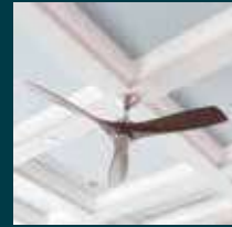
CEILING ACRYLIC EMULSION PAINT/ OIL BOUND DISTEMPER
