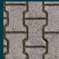
INTERNAL ROADS INTERLOCKING BLOCKS/ TREMIX CONCRETE ROAD
